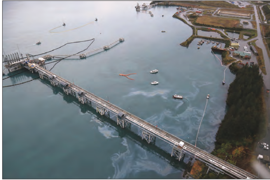
The Sept. 21 spill at the terminal was what Alyeska described as “oily test water” believed to have resulted from flow back during a test of the integrity of the loading arms.
