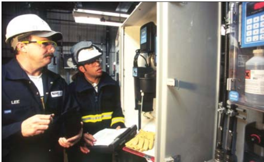
Two NANA/Colt designers check out the equipment at the Alpine field wastewater plant
