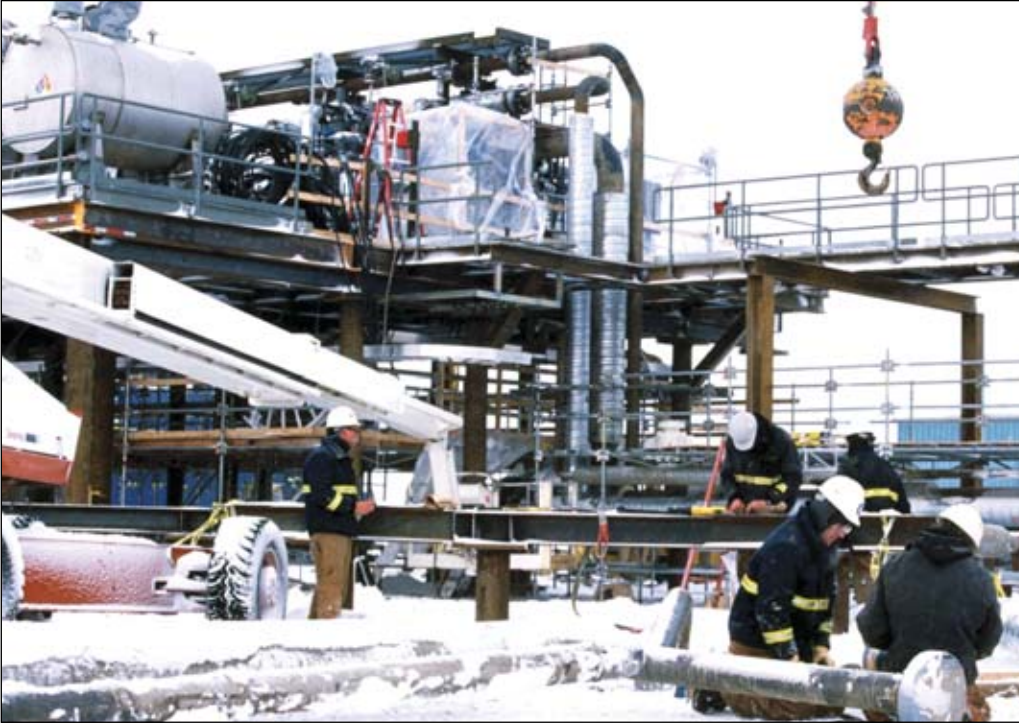
Above, staff on site to assist the construction crew during installation of new Prudhoe Bay WRD facilities that were engineered and designed by NANA/Colt. At right, The Arctic Millennium's Tundra Track exerts only 55 psi loading pressure on the tundra. The track-mounted rig can deliver cost effective and technologically superior drilling capabilities to remote locations.
