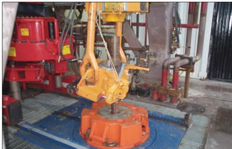
The Arctic Millennium's automated pipe handling increases rig safety.
