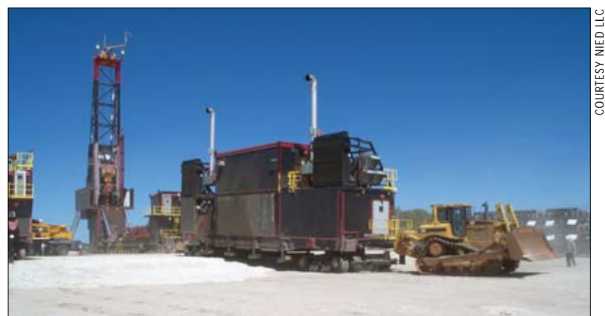
Moving the Millennium's power module.
