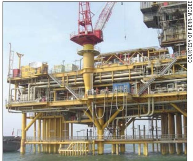
This wellhead gathering platform (WGP-A) is part of Kerr-McGee's new core operating area in Bohai Bay, China, which includes two platforms and one large throughput floating production, storage and offloading facility.
