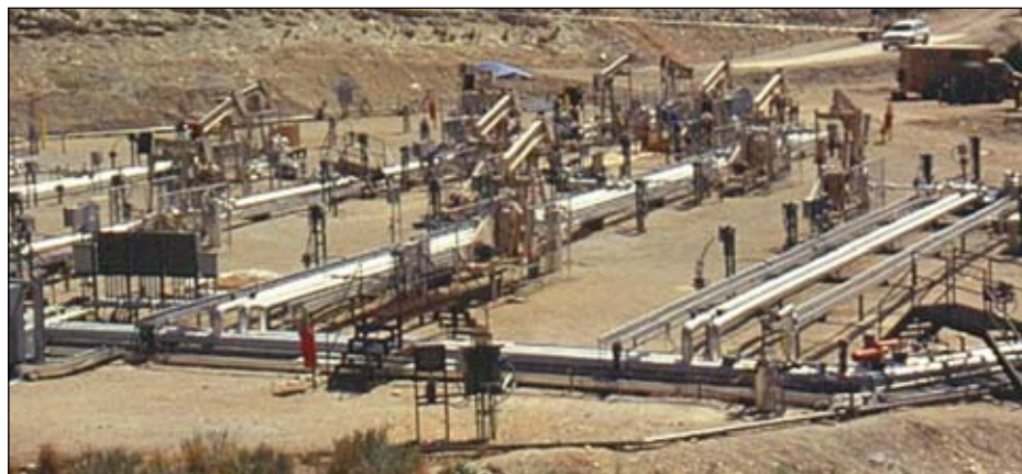
Shell's ICP shale oil layout resembles an oilfield production complex typical of those found in Colorado's conventional "oil patch." Some piping carries condensed shale kerogen from heated well bores to processing facilities, while others are used to surround underground well bores with an "ice barrier."
