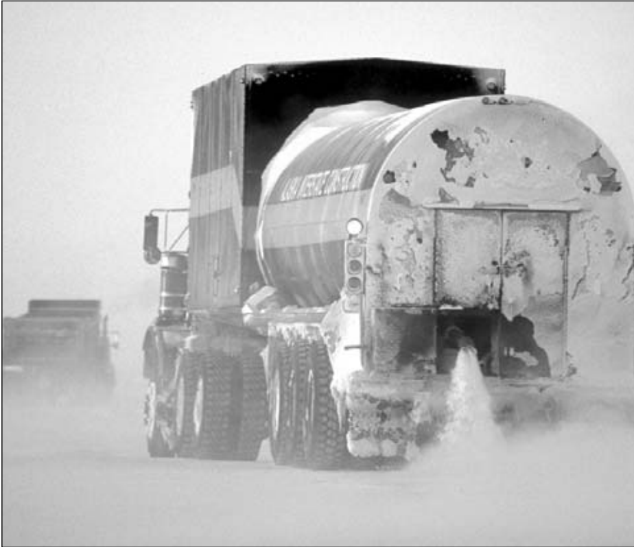
An AIC water tanker applies water to an offshore ice road under construction. The ice road and ice islands were built to support the offshore exploration for Pioneer Natural Resources and Armstrong Oil and Gas during the winter of 2003.
