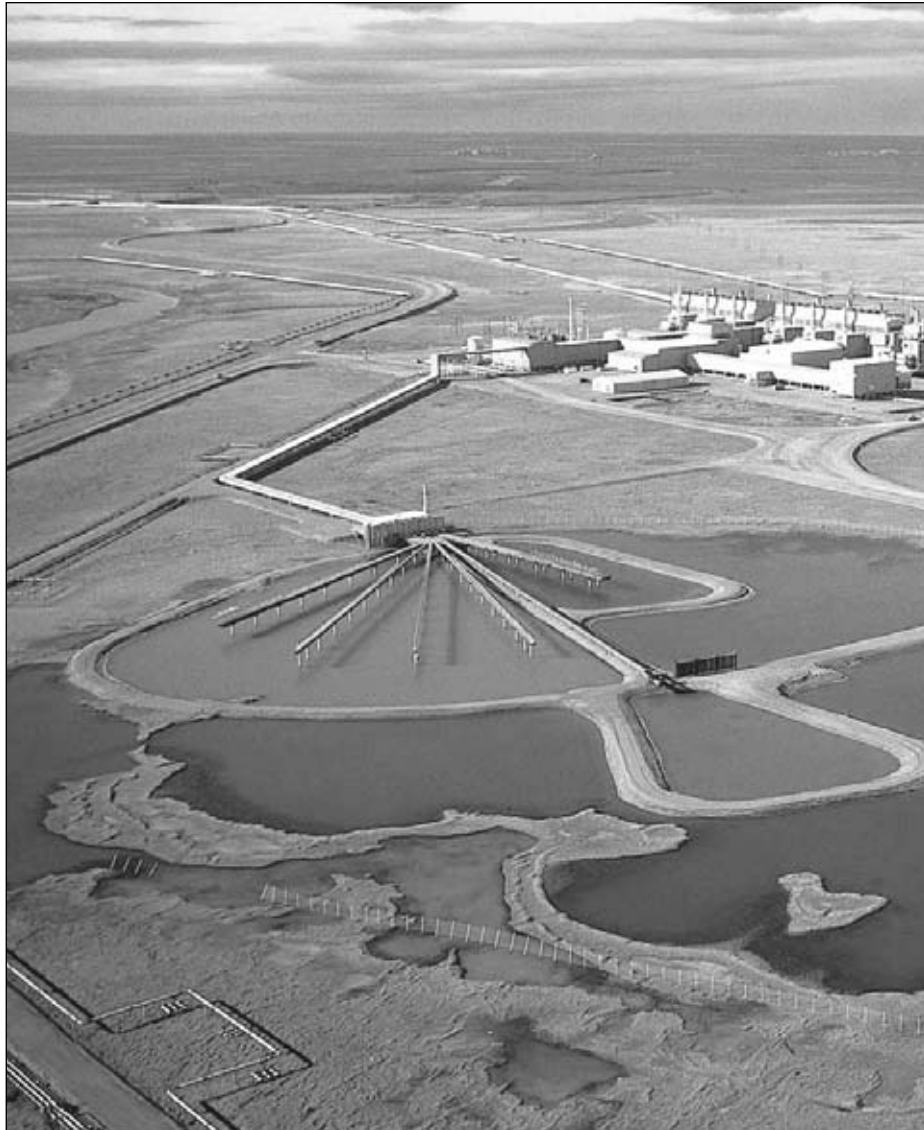
Gas is currently reinjected at the giant Prudhoe Bay field on Alaska's North Slope. Above photo is the BP-operated gas injection facility at Prudhoe.
