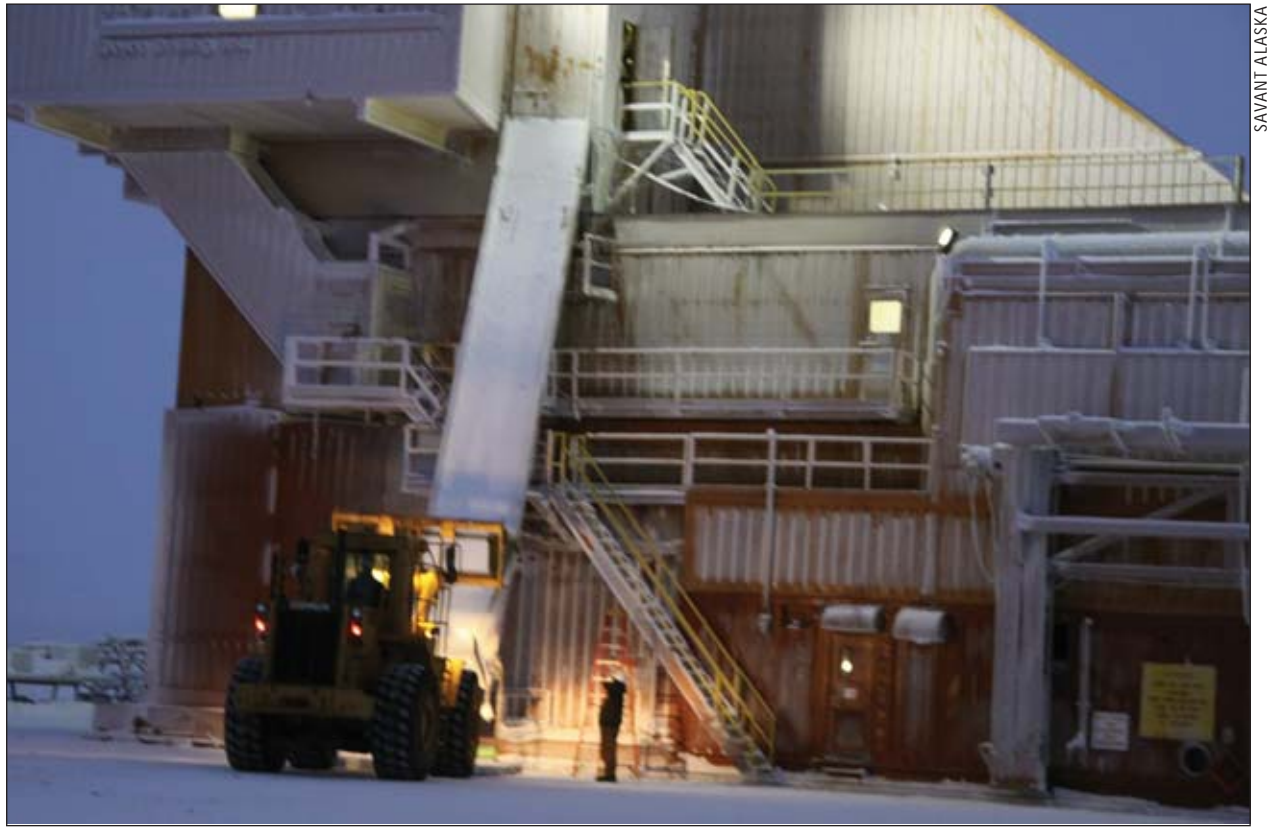
Doyon Rig 15 at Deadhorse on Alaska's North Slope.
