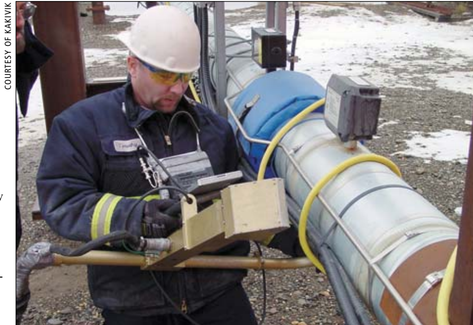
A Kakivik inspection technician works with a C-Arm or CUI System.
