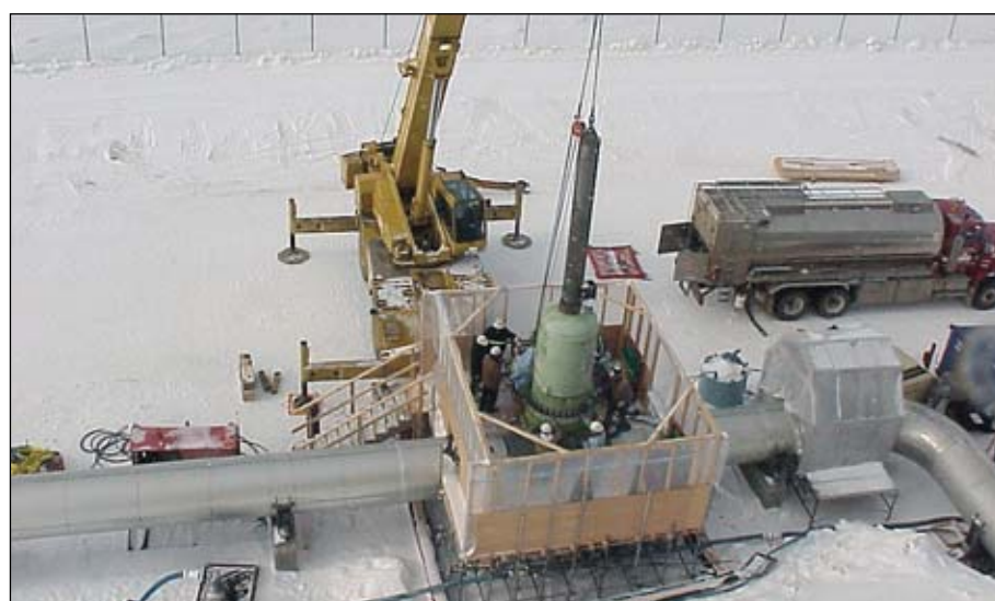
Installation of a remote activated gate valve
