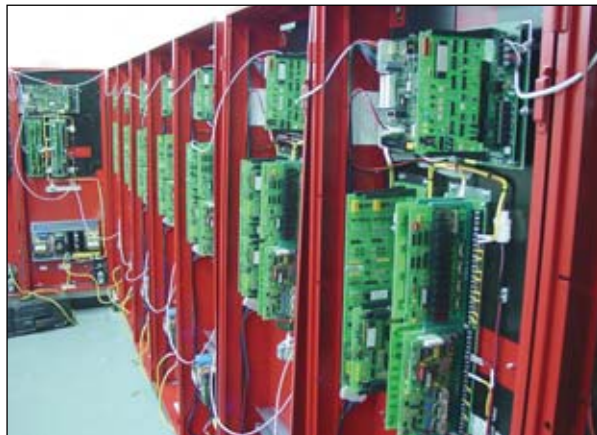
In the fabrication shop at Engineered Fire and Safety, these fire alarm control panels are being fabricated for the Basset Hospital at Fort Wainwright, Alaska.
