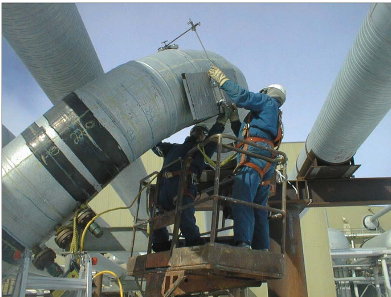
Kakivik Asset Management workers prepare a TRT film setup for an inspection. Analysis of the data from the inspections provides insights into how to manage a corrosion control program — the purpose of the inspections is to help customers identify problems well before the corrosion threatens the integrity of a facility. See Kakivik's company profile on page B13.
