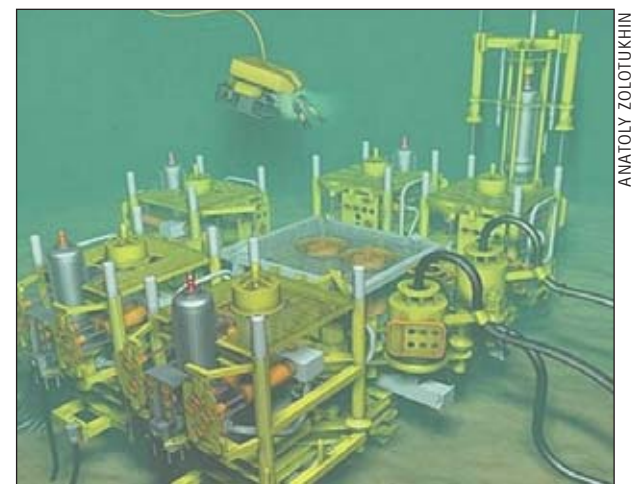
At left, the Åsgard field floating production and accommodation facility uses a ship stationed over a vertical turret containing the well risers. At right, is this the offshore oil field of the future? — a subsea production facility remotely controlled and maintained from land.
