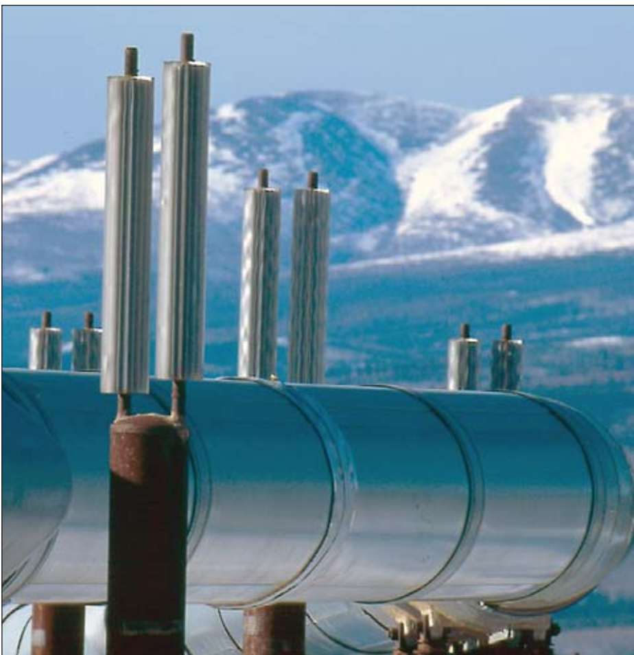
The 800-mile trans-Alaska oil pipeline runs from Prudhoe Bay to the Port of Valdez.
