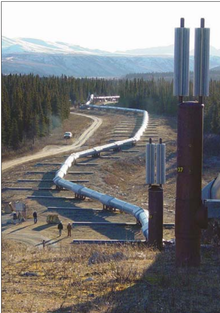
Michael Baker's pipeline expertise was called upon within hours of the November 2003 earthquake near Delta Junction, Alaska. Although the Trans-Alaska Pipeline performed as designed, it did sustain some damage to the above ground support system. The company is completing a corrective redesign to be implemented this summer.
