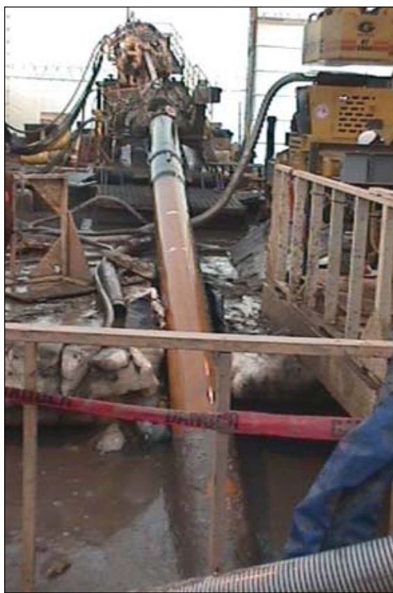
For designing the first horizontal, directionally drilled pipeline in the Arctic, Michael Baker Jr. received the Alaska and Northwest District Civil Engineering achievement of the Year award in 1999 for the section of the Alpine pipeline that passes under the Colville River.
