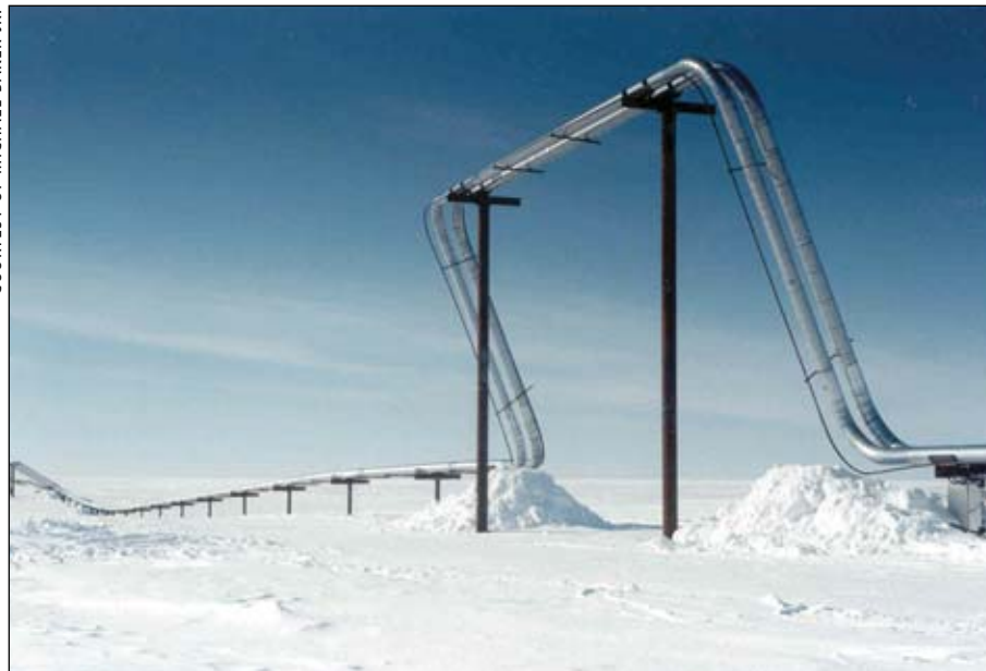
Developed at Michael Baker Jr. for the Alpine project, the innovative vertical loop concept sets up artificial terrain breaks that create a spill isolation function superior to valves.
