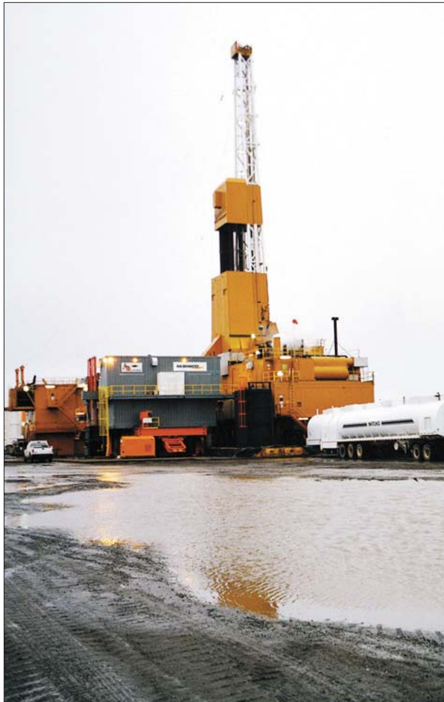
The M-I SWACO cuttings grinding and injection unit at the Alpine field continues to roll up milestones.
