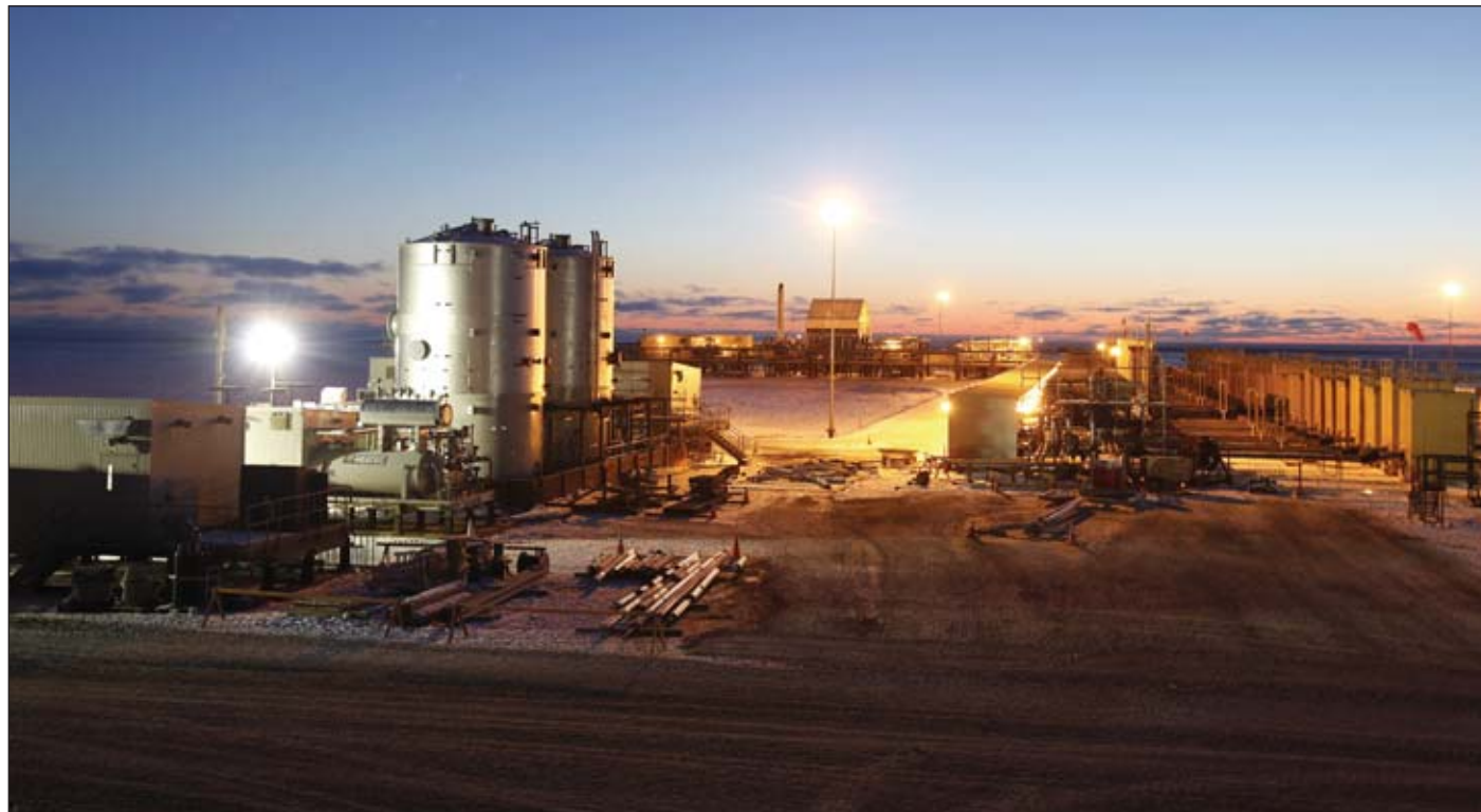
BP's new heavy oil test production facility, seen on the left side of this recent photo of the Milne Point S-Pad on Alaska's North Slope, should go into operation in May. The two large, cylindrical tanks in the center of the facility will separate sand from the heavy oil, pumped as an oil and sand slurry from the Ugnu formation 4,000 feet below the pad.
