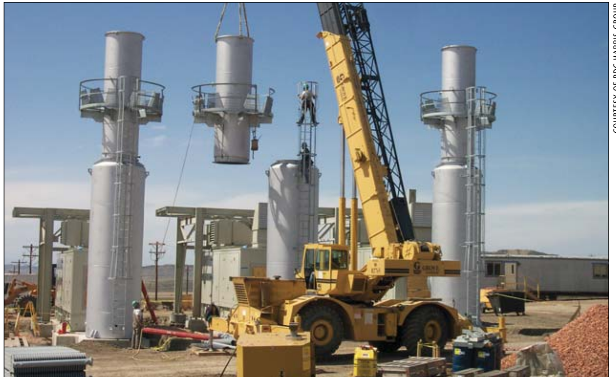
Simple cycle gas turbine electric power generating station engineered by PDC Harris Group.
