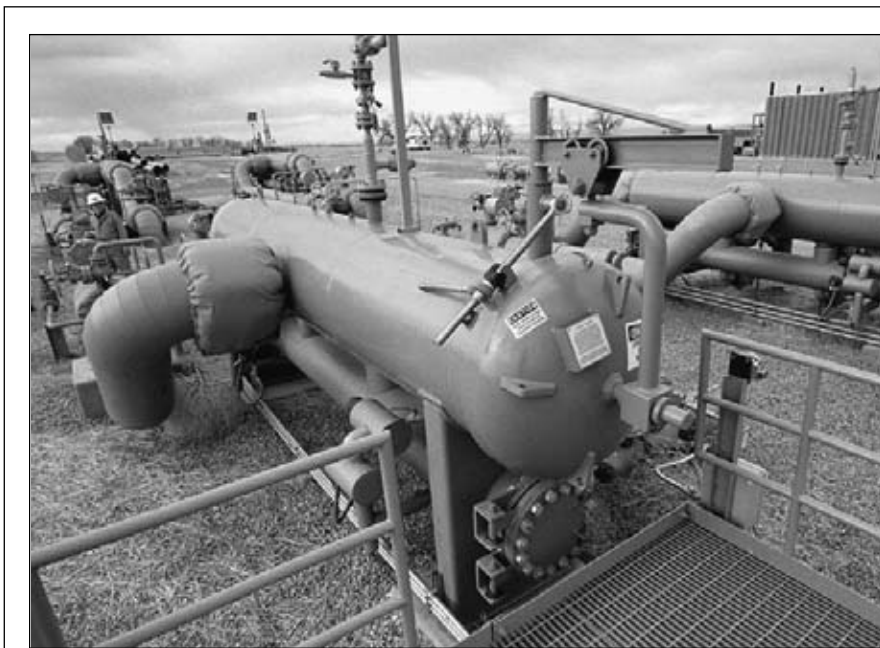
Pig barrel, Fort Lupton, Colo. Engineering and design by PDC Harris Group. See the company profile on page B12.
