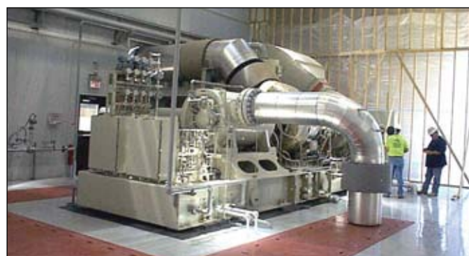
Natural gas compressor station engineered by PDC Harris Group.
