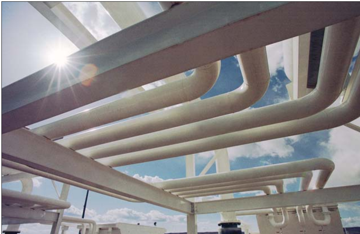
An overhead pipe rack engineered by PDC Harris Group at the Rawlins Jumper Compression Station in Rawlins, Wyo.
