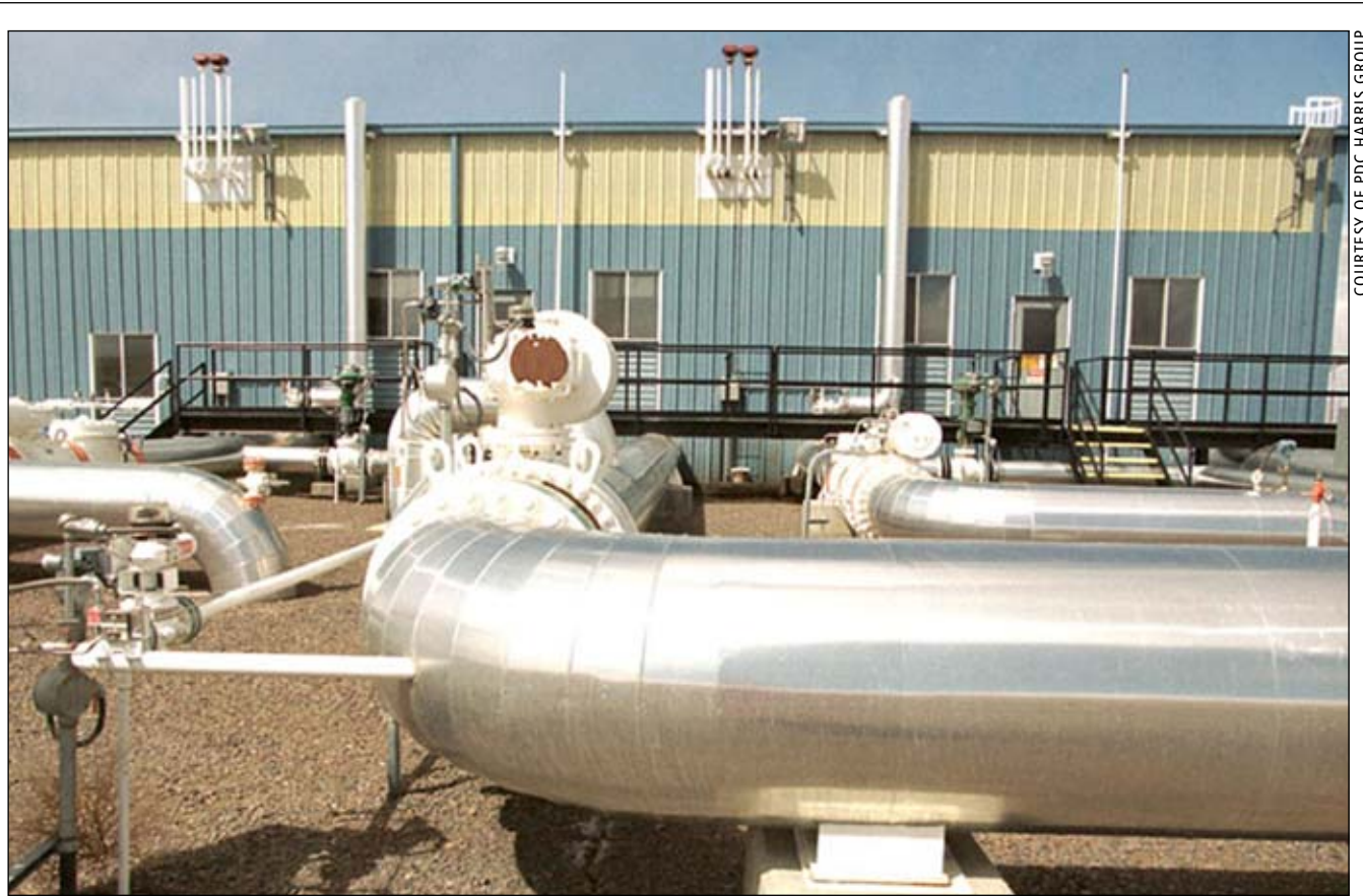
Inlet gas piping entering a compressor station building in Laramie, Wyo. PDC Harris Group was part of the project design. See the company profile on page B12.
