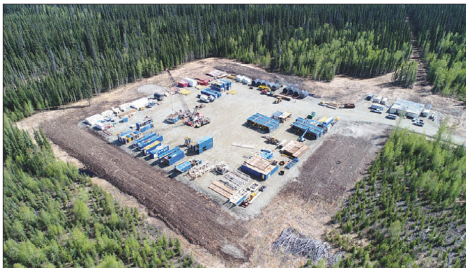
In the winter of 2017-18 Doyon Ltd. constructed the gravel pad for the drilling of the Totchaket No. 1 well. A short gravel access road linked the pad to the nearby Tanana River for transportation to and from the drill site.
