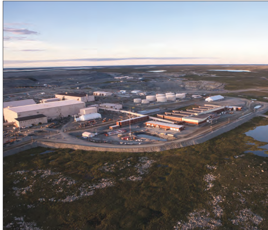
Since going into production in 1998, the Ekati diamond mine in Northwest Territories has become world-renowned for its premium diamonds. A recent fire in the processing facility is expected to curtail the production of these gem-quality diamonds in 2016.
