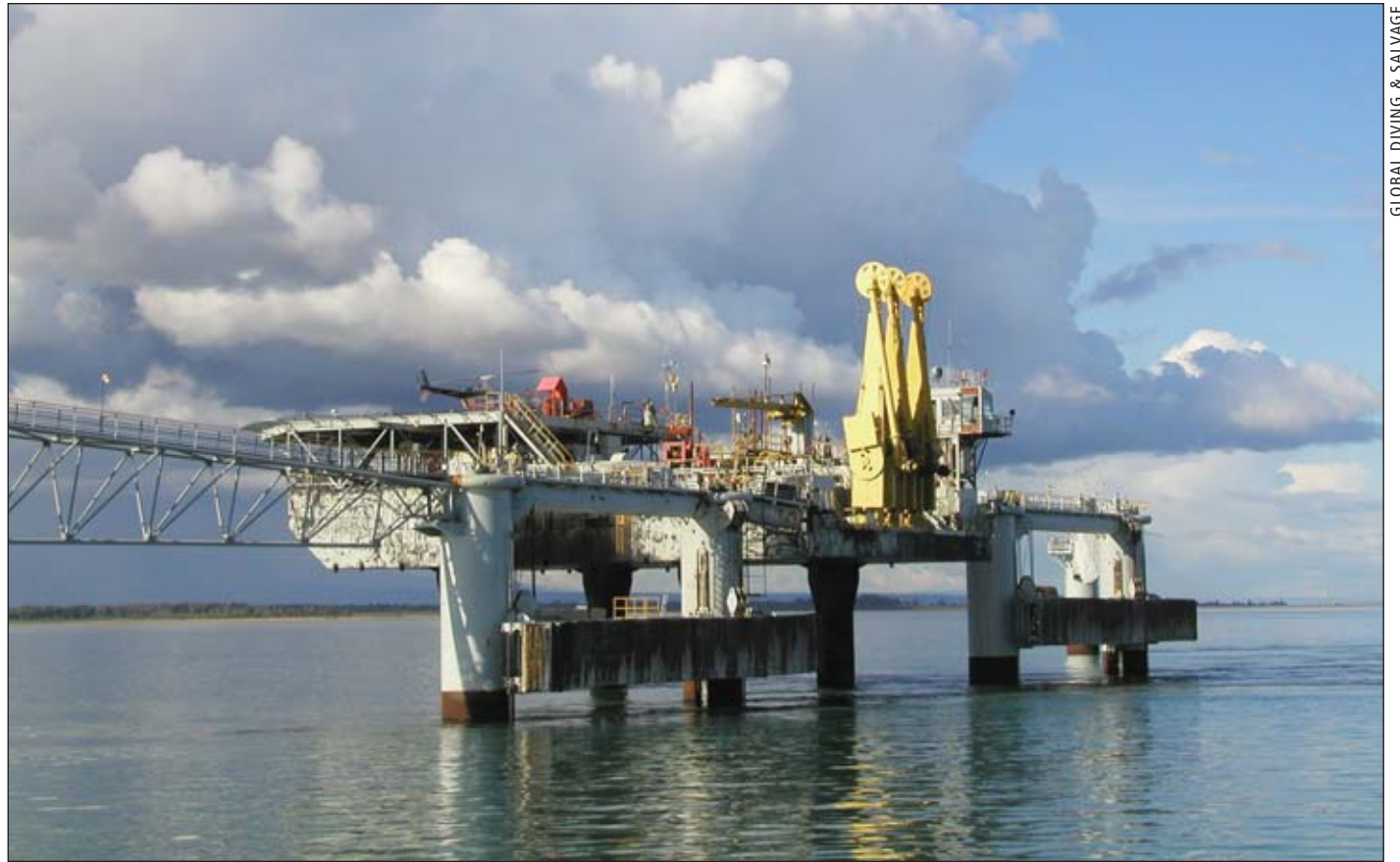
A mechanical failure caused a fender on the Christy Lee loading platform to fall into Cook Inlet. The fenders are the large, flat pieces visible here. Tankers lay against the fenders while docked to load crude oil.
