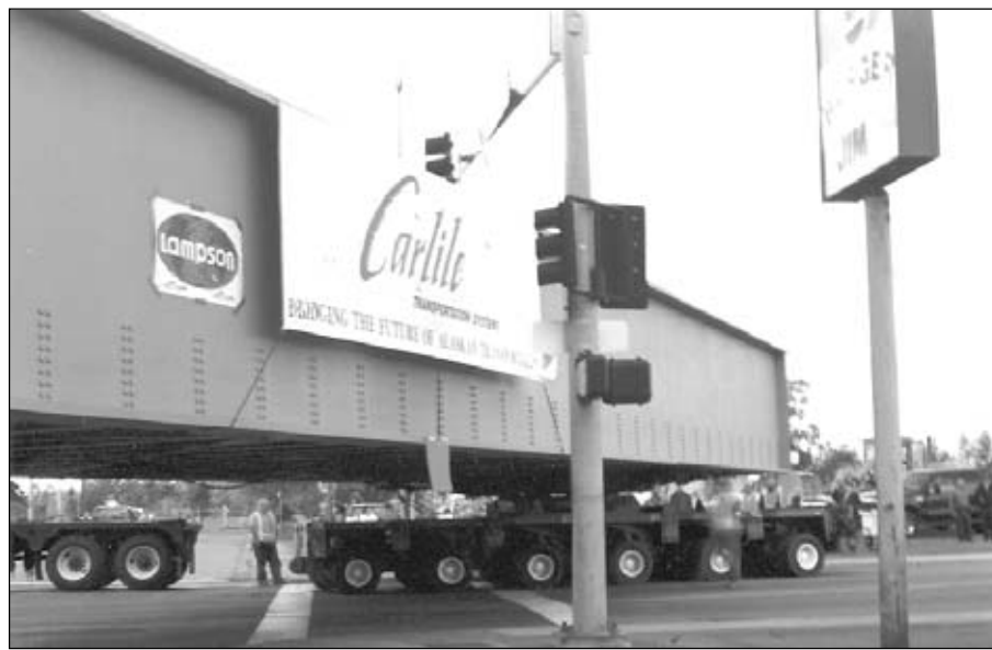
The bridge for Alaska Railroad's airport terminal rounding the corner at 4th Avenue and Gambell Street.
