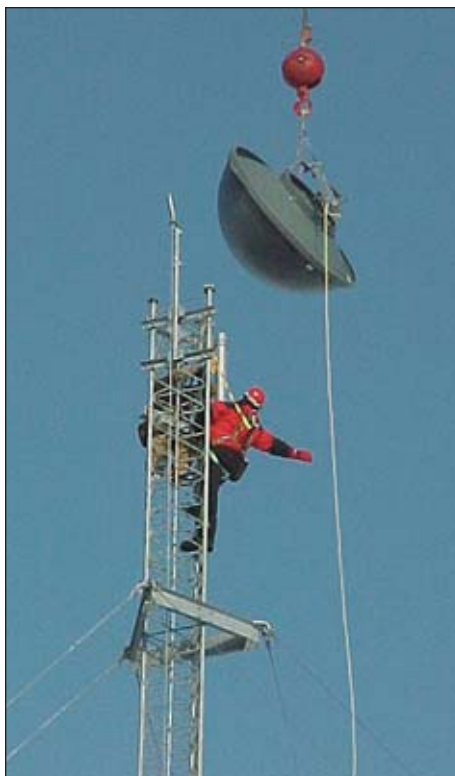
Installing a microwave radio antenna during the Alpine project.
