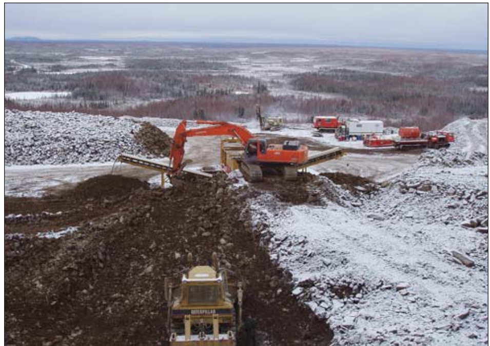
Cruz Construction's rip-rap plant in operation
