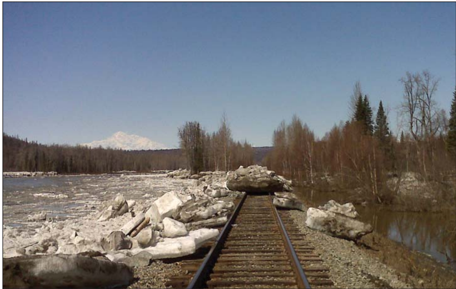
The Alaska Railroad’s 500 miles of track sometimes sustains damage from melting snow and ice during breakup. Ice and gravel cover these tracks that washed out during spring flooding in May. Much-needed federal funds help to cover the cost of annual repairs to the railroad’s more than 500 miles of track.
