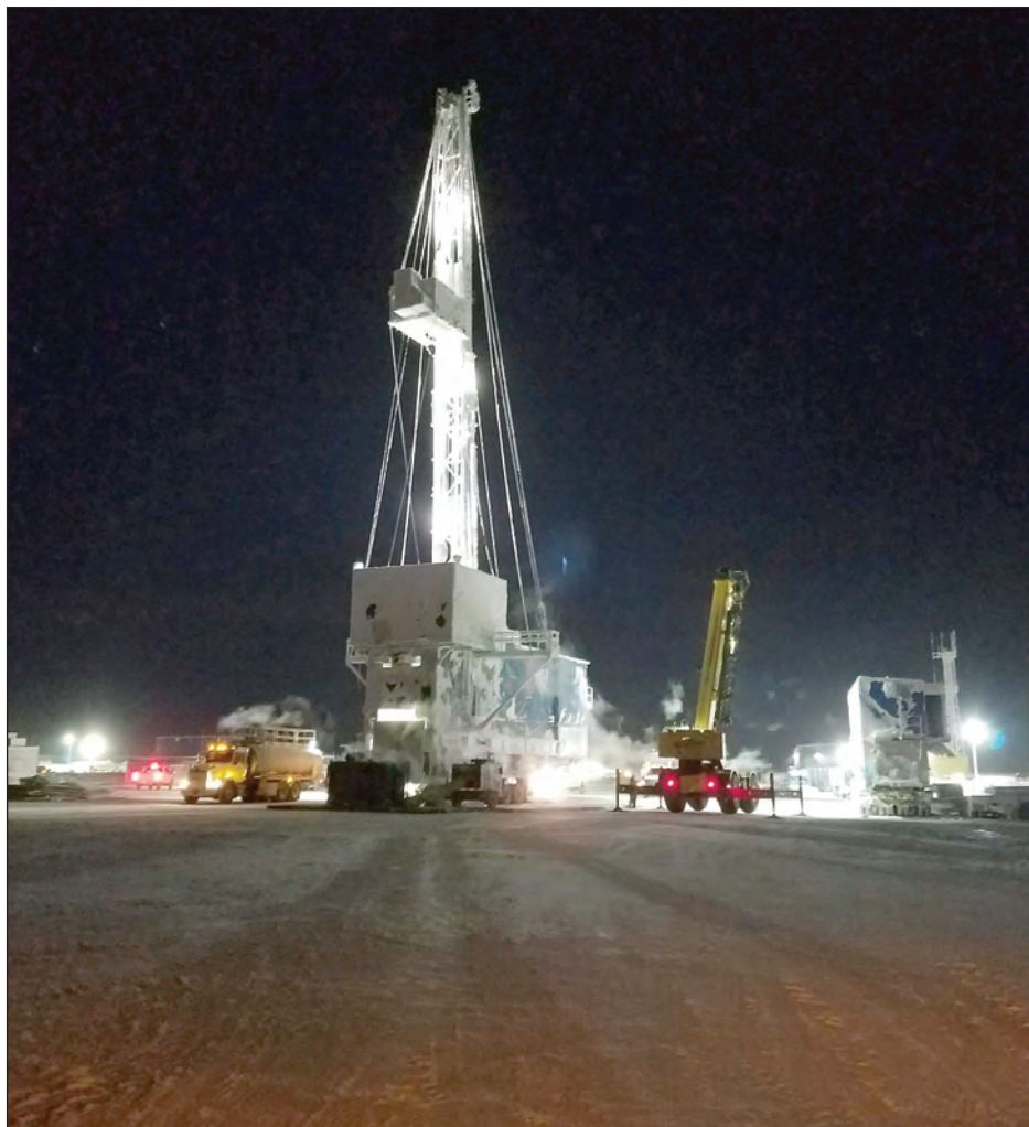
Rig-111 commissioning work, January 2021
