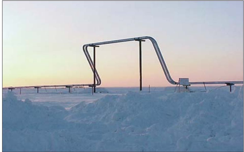
Alpine Pipeline Vertical Loop. Vertical loops create artificial terrain breaks and form a terrace structure. They work by creating hydraulic break points in the pipeline, performing a spill isolation function superior to valves. The design breakthrough not only saved money, it set a new standard for pipeline integrity. Vertical loops were reviewed and approved under a waiver granted by DOT.
