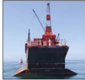
The SDC — i.e. steel drilling caisson — a bottom-founded Arctic drilling platform, managed by Fairweather E&P Services.
