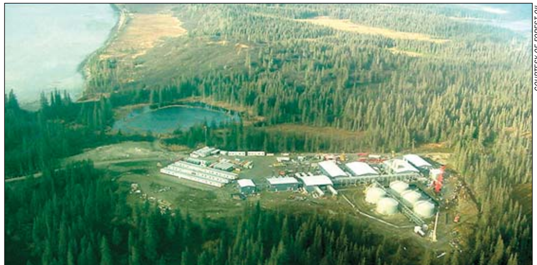
THE KUSTATAN PRODUCTION FACILITY AND CAMP FOR THE REDOUBT SHOAL UNIT DEVELOPMENT.
