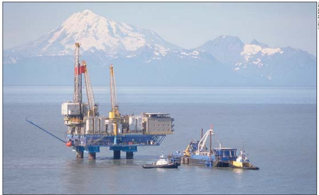
Redoubt's Osprey platform was the first platform to be set in Cook Inlet since 1986. The 3,200-ton platform was designed to withstand winds of 140 miles per hour and cost $30-$35 million to construct and set in place. The cost does not include the pipelines. The platform has 28 slots; 15 dedicated to oil producers, three to gas, and 10 will be for water injectors for pressure maintenance.
