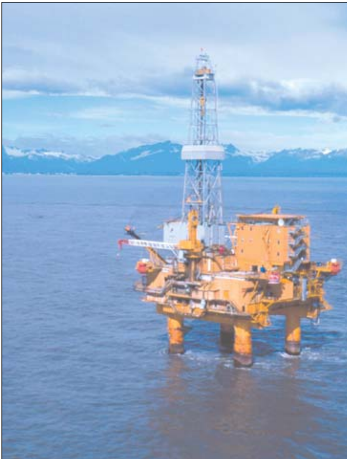
An XTO platform in Cook Inlet
