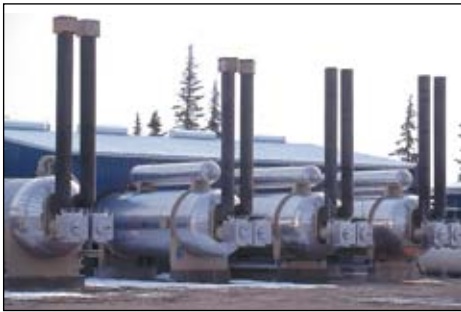
A closer look at Forest's Kustatan production facility
