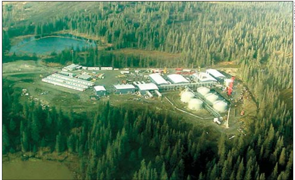
An aerial view of the Kustatan production facility and camp for the Redoubt Shoal unit development.
