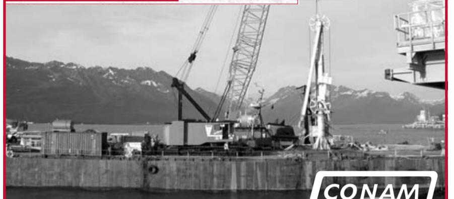
Replacing Alyeska's Oil Tanker Loading Arms
