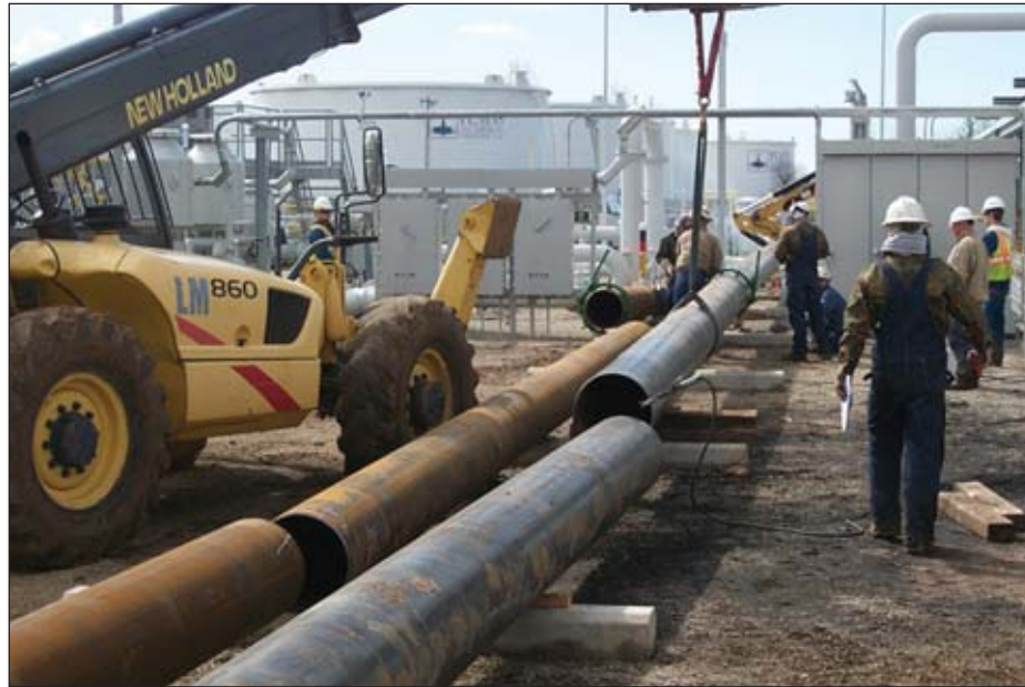
Above, workers prepare for the first weld at the Cushing station in March. Below, a section of pipe is lowered into place
