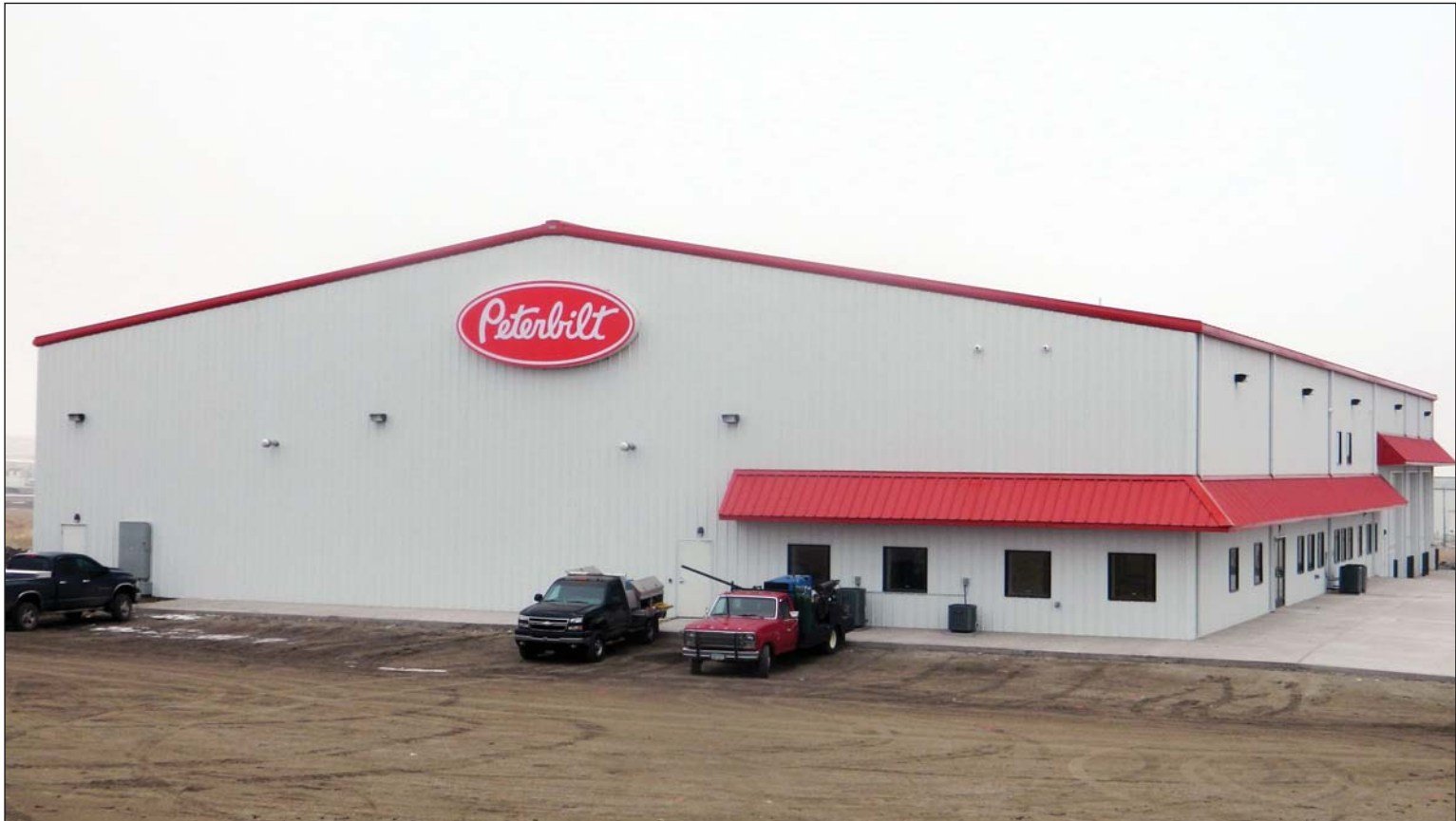
Allstate Peterbilt of Williston's new full-service facility
