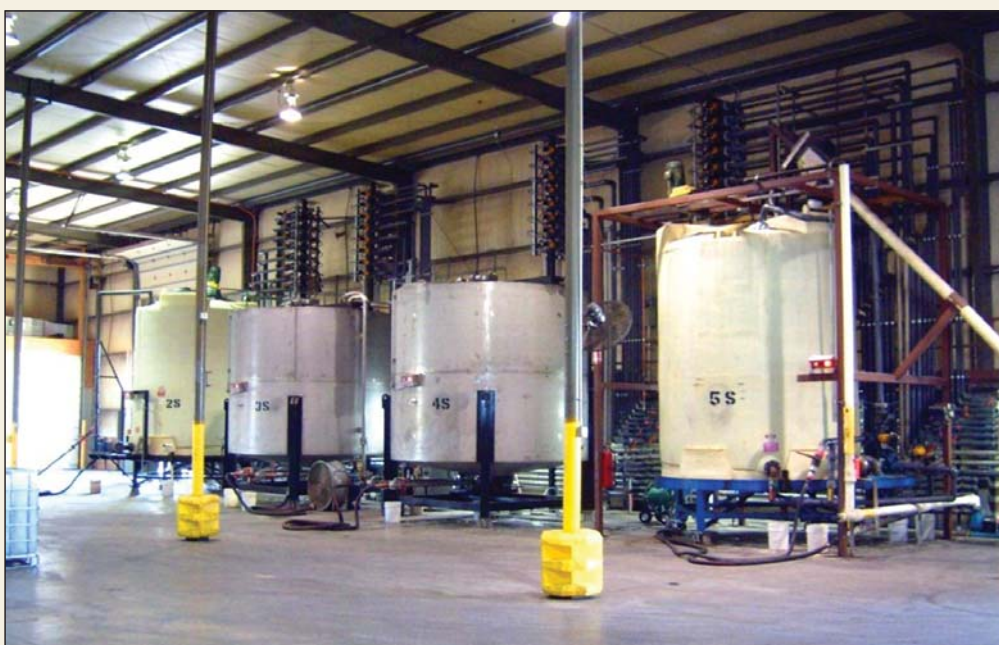
CESI's new 8,000 gal stainless steel liquid blend tanks
