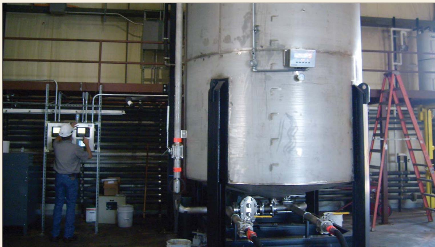
CESI's new 8,000 gal stainless steel liquid blend tanks
