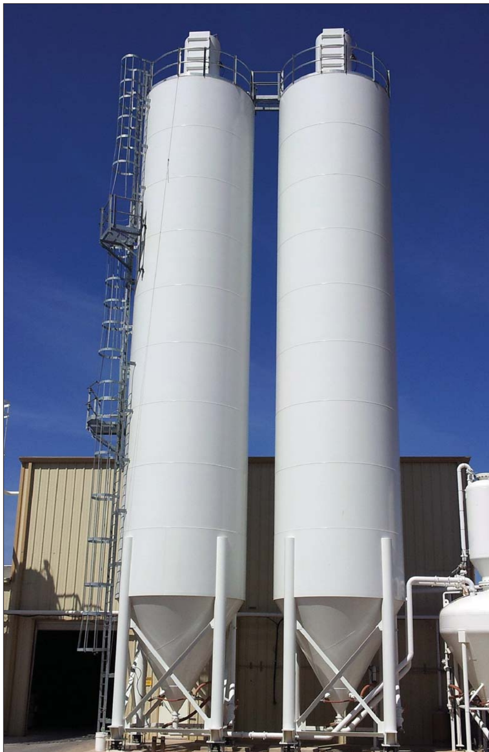
Dry chemical storage tanks at Marlow facility. Photo by CESI Chemical, Inc.
