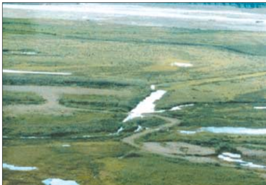
Pictured here is the northern end of the Umiat Airstrip and the gravel road that leads to the Seabee well site. The Colville River is in the background.
