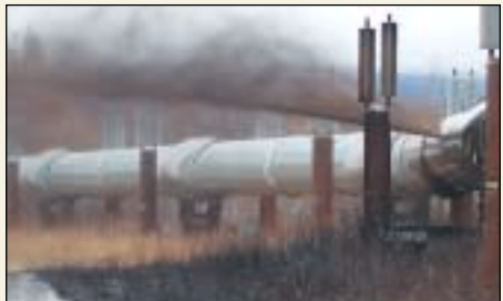
Some 6,800 barrels of Alaska North Slope crude hit the ground about 45 miles north of Fairbanks between the time a bullet punctured the trans-Alaska oil pipeline at about 3 p.m. Oct. 4 and 3 a.m. Oct. 6 when a hydraulic clamp sealed off the spill.
