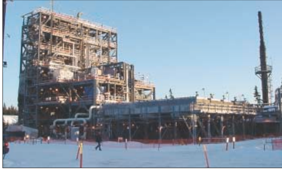
BP's GTL plant under construction in Nikiski. Photo taken Feb. 12.
