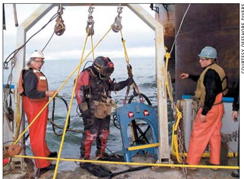
On the deck of the Sand Island, inside the A-frame. The diver used the blue pipe-cutting saw to sever an oil pipeline running to the Cook Inlet platform visible on the right. After cutting the line, divers attached a flange and connected it to another pipeline.
