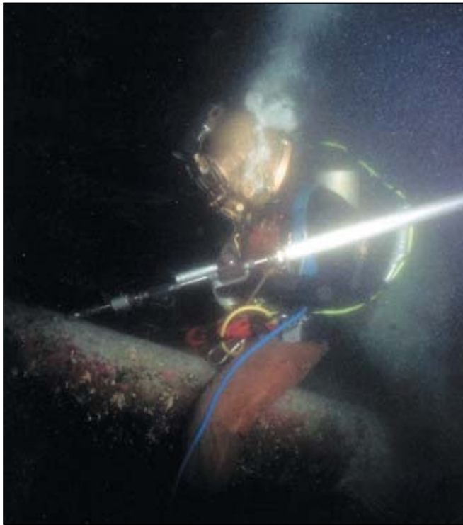
Diver Tobin Frey water blasts a horizontal member on a loading dock structure at the Valdez tanker terminal.
