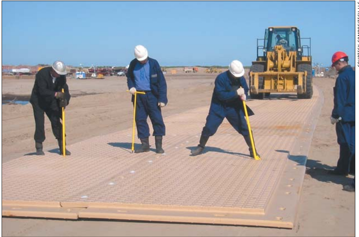
Fastening mats on a temporary road on Sakhalin Island
