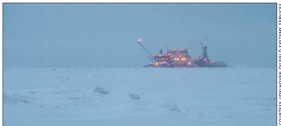
Udelhoven Oilfield Systems Services, one of Alaska's premier oilfield service companies, uses First National Bank financing to help it provide responsive services that include construction management, quality assurance and functional checkout at BP's Northstar oil platform. Through First National, Udelhoven and other oilfield service companies finance projects, equipment and services.
