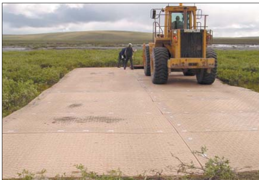
Installing a temporary road for a project on the trans-Alaska pipeline
