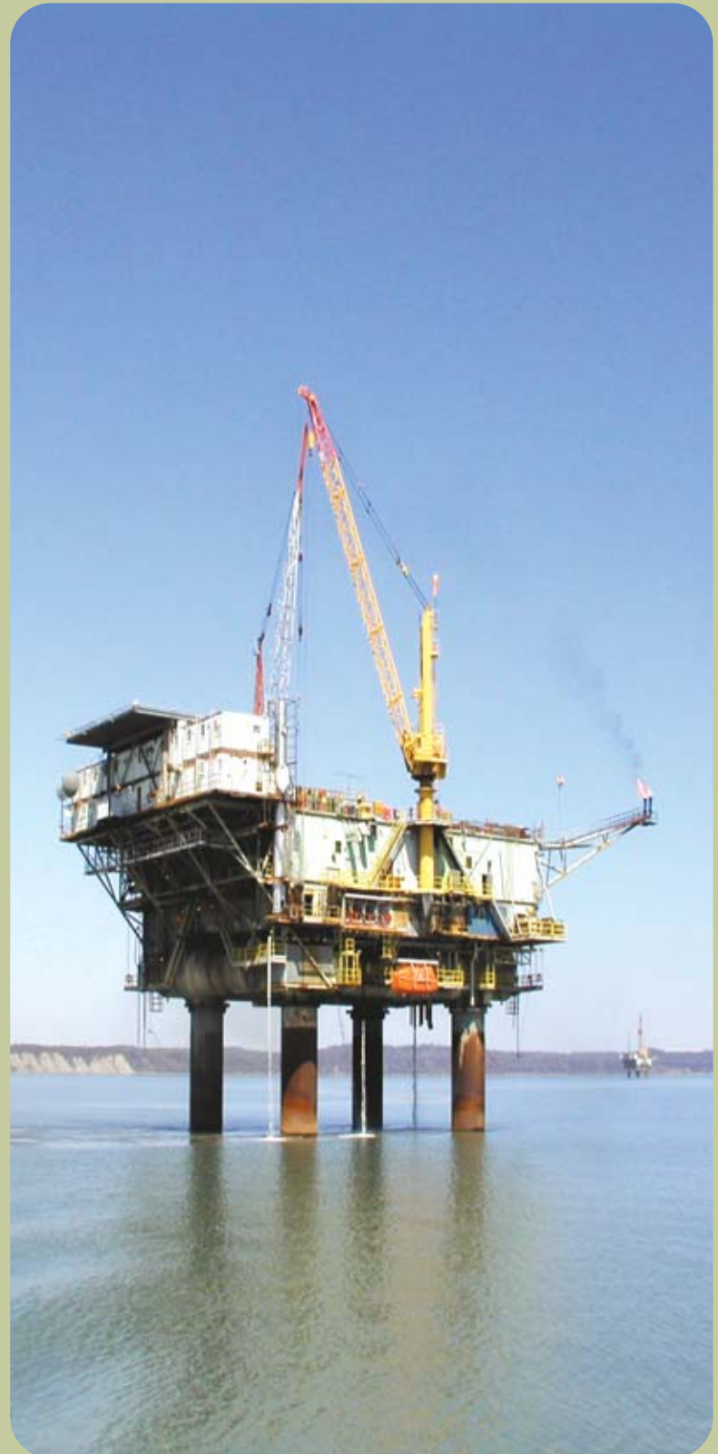
Cook Inlet Platform
