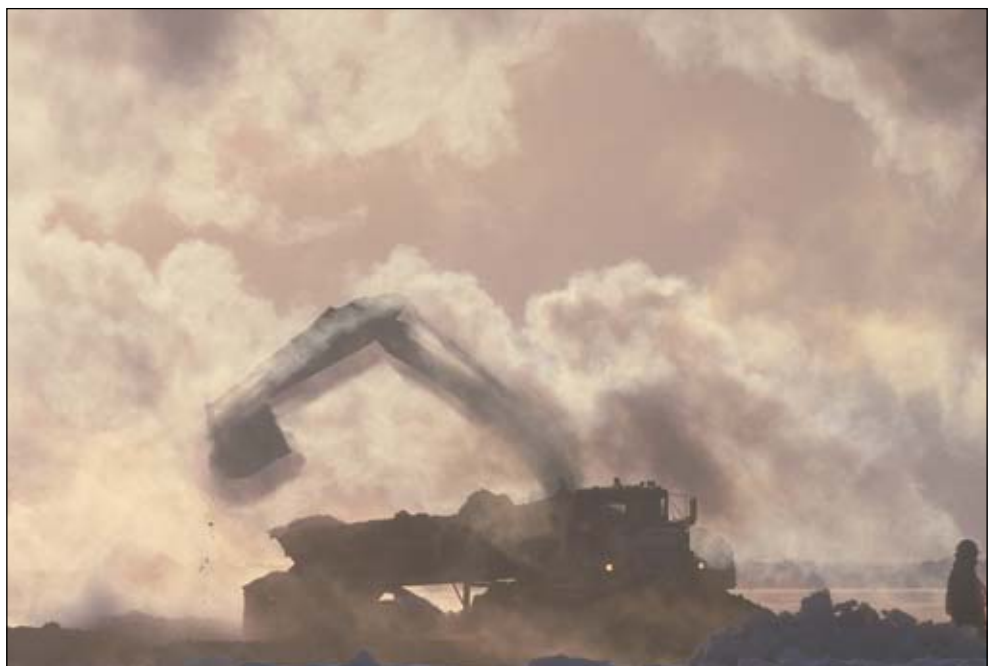
Backhoes excavating ice during Northstar Island construction
