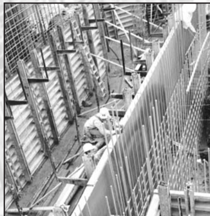
Bradley Lake Hydroelectric Project. Homer, Alaska
