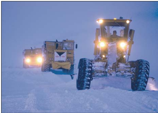
Ice road construction on the North Slope
