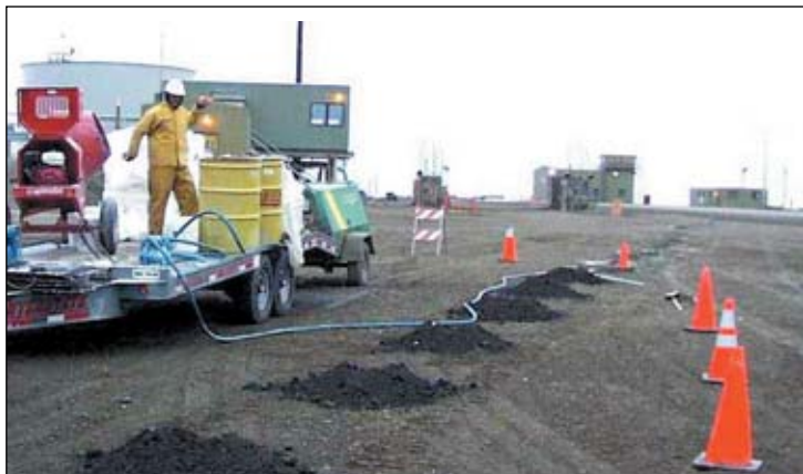
ENSR workers pump an oxygen-releasing compound slurry for enhanced aerobic bioremediation at a North Slope site.
