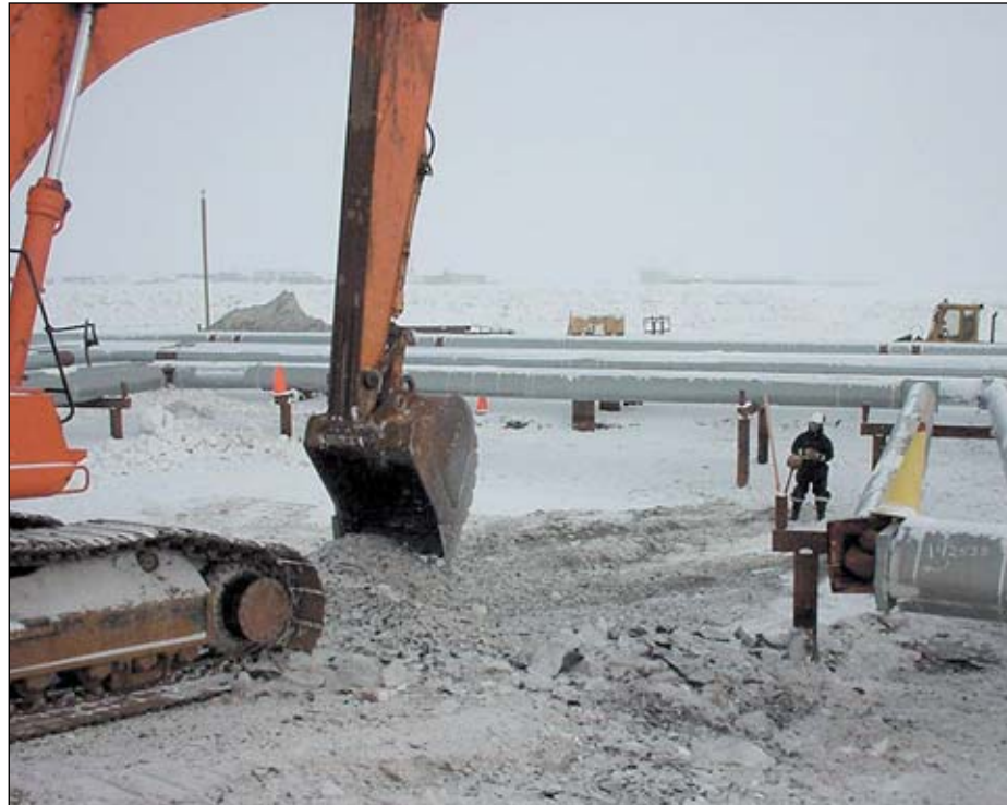
Excavating contaminated material at a spill site on the North Slope
