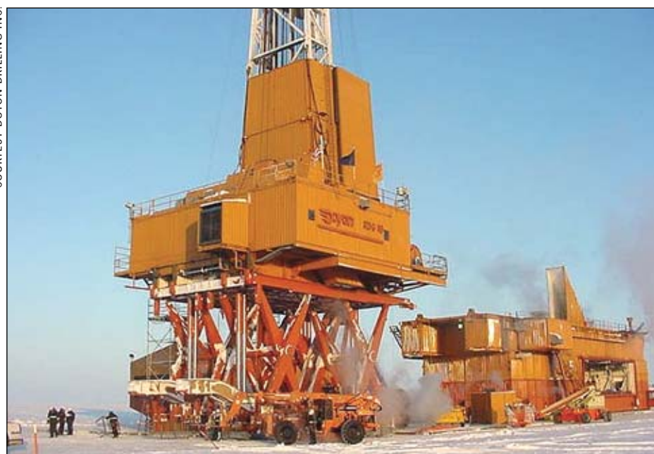
A unique scissors mechanism lifts Doyon Drilling's Rig 19 rig floor and derrick onto a transporter.
