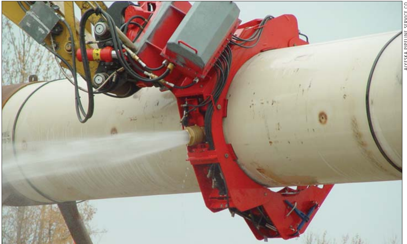
Alyeska Pipeline Service Co. teamed with Fairbanks firms, Mustard Engineering and Holaday-Parks metal shop to design and build the HC 320 Hydraulic Clamp after the Milepost 400 bullet-hole incident in 2001. Once applied to the trans-Alaska oil pipeline as a temporary patch, the clamp can be left in place. This allows Alyeska to deploy multiple clamps, if needed.
