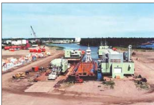
Loading the modules for the Badami field at Northern Transportation's Hay River terminal
