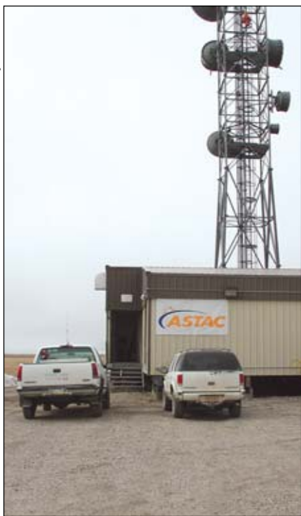
ASTAC's central office in Deadhorse is topped by a state-of-the-art microwave tower.
