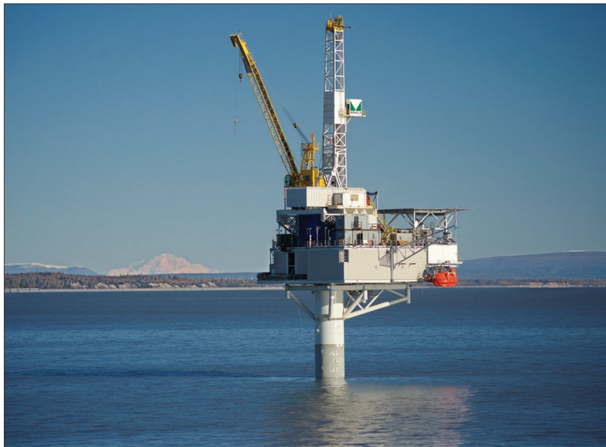
Julius R. production platform with Denali in the background.
