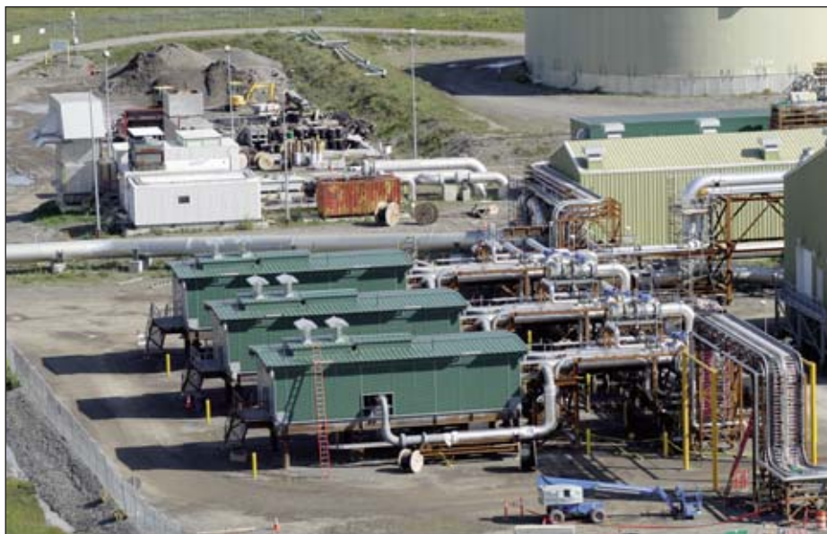
Located in the foothills of the Brooks Range, pump station 3 was the second pump station to begin using new electrical pumping equipment and control systems. The green buildings in the foreground house the new pumps.
