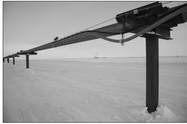
By building a 70,000 barrel per day liquids export pipeline at Point Thomson that connects to the Badami unit and thus moves oil and condensate to Pump Station 1 of the 800-mile trans Alaska oil pipeline, ExxonMobil improved the development economics of other oil prospects to the east, including Sourdough and Yukon Gold. Production from Point Thomson continues to remain around 10,000 bpd.
