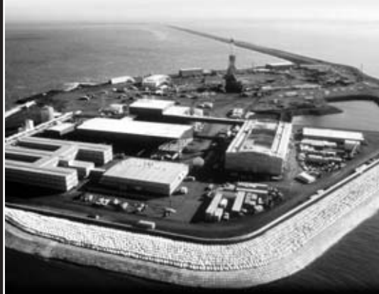
Workforce Housing, Prudhoe Bay, Alaska
