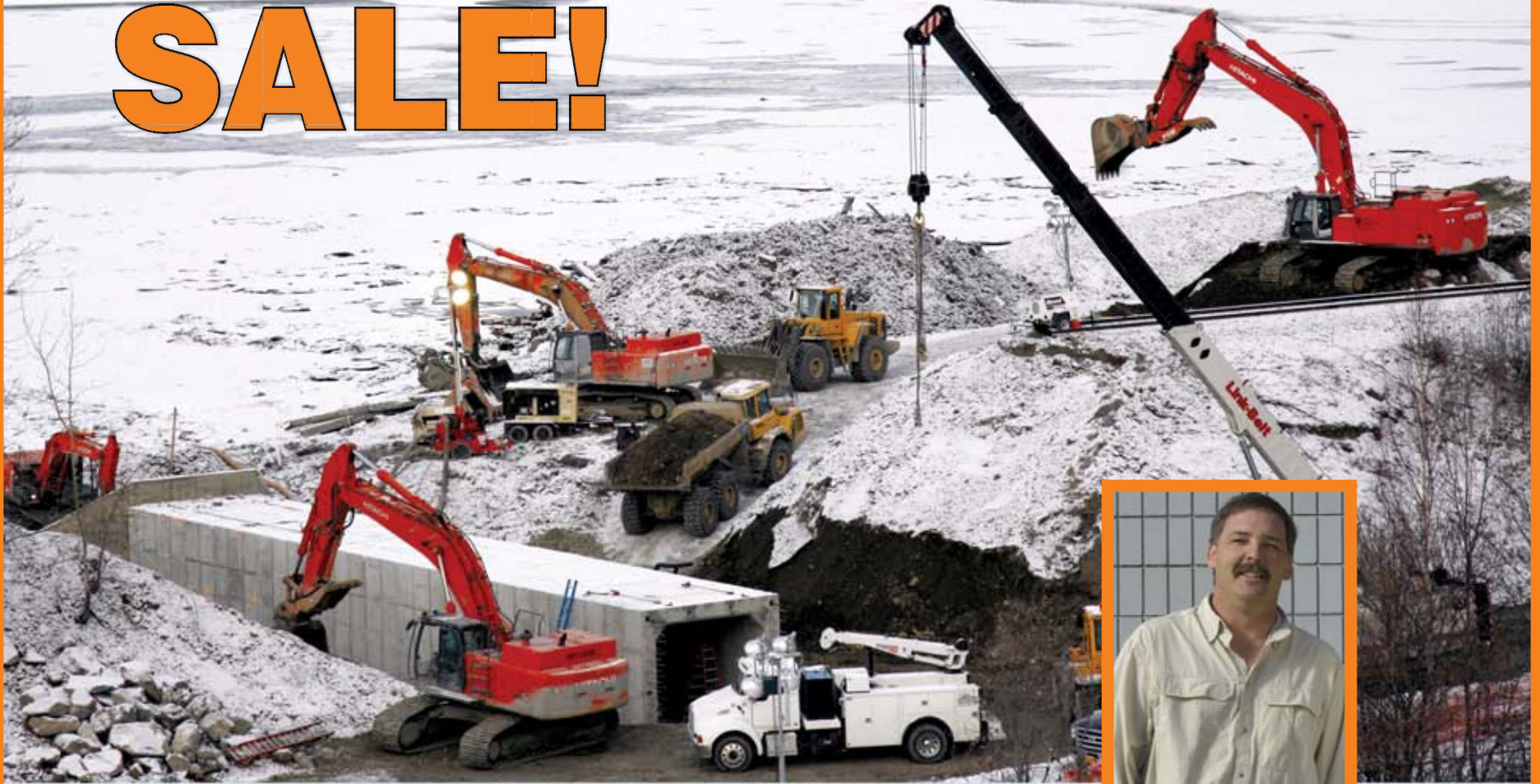
Above photo: Volvo, Hitachi, and Linkbelt equipment at the Hamilton Construction job site, Chester Creek, Anchorage
