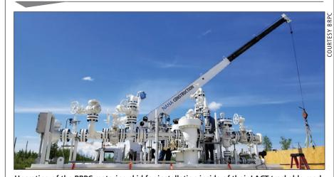
Uncrating of the BRPC metering skid for installation inside of their LACT trackable module at Mustang, courtesy of NANA Construction's Big Lake fabrication facility.
