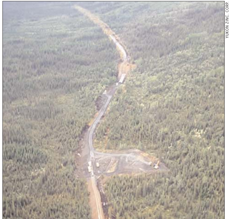
An aerial view taken July 30 of the 15-mile access road under construction this summer, linking Yukon Zinc Corp.'s Wolverine project with the Robert Campbell Highway in Yukon Territory.
