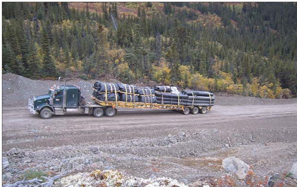
Large trucks are now able to transport equipment and supplies to the remote Wolverine project thanks to this gravel access road. Workers nearly finished the artery this season. The project is poised for a production decision in October, once financing is completed. Startup is envisioned for early 2009.
