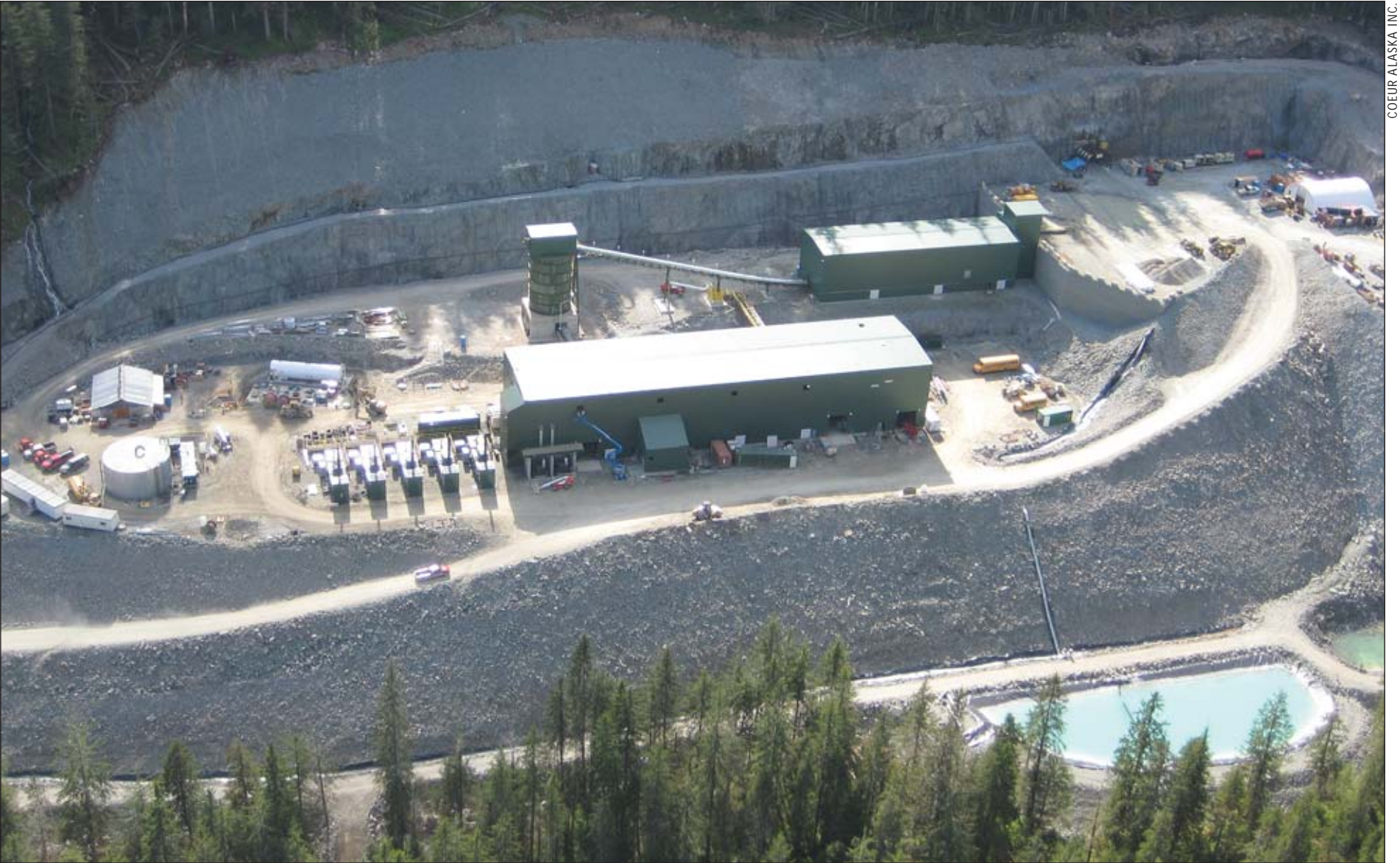
An aerial photo of the newly completed mill site at the Kensington Gold Mine shows generator-sets, mill and crusher buildings as well as the Jualin portal.
