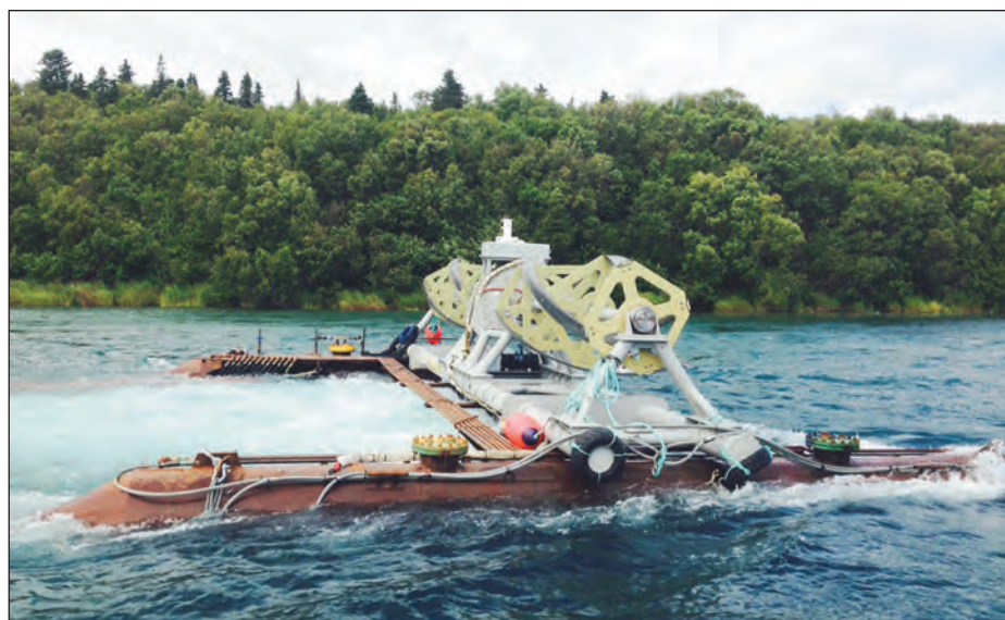
Ocean Renewable Power Co.'s RivGen being deployed in the Kvichak River during the summer. The device was sunk to the bottom of the river, enabling its helical shaped turbine to generate electricity for the village of Igiugig.
