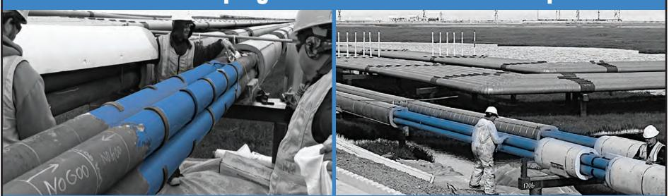
Polyguard Products has introduced a really different type of corrosion protection to address Alaska's corrosion problems. ReactiveGel® (nicknamed "BlueGoo®" by Oil Patch users) is a patented product which reacts with steel surfaces to form a microscopically thin glasslike surface. This glasslike surface will not corrode.
