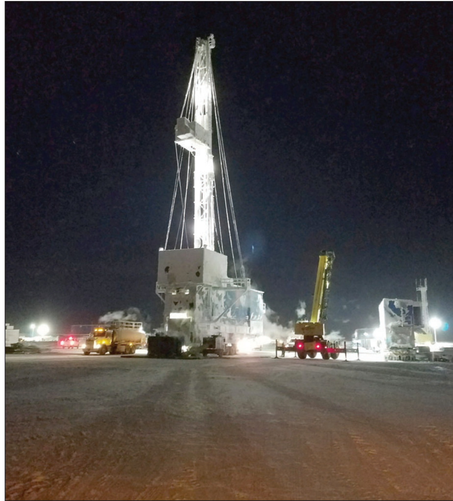
Rig-111 commissioning work, in January 2021 for Merlin 1.
