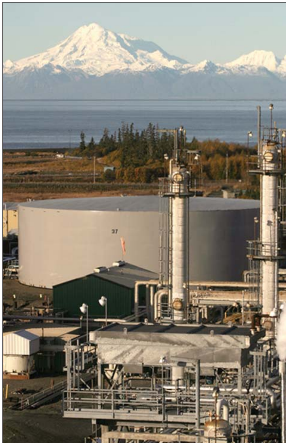
Tesoro's Nikiski, Alaska refinery
