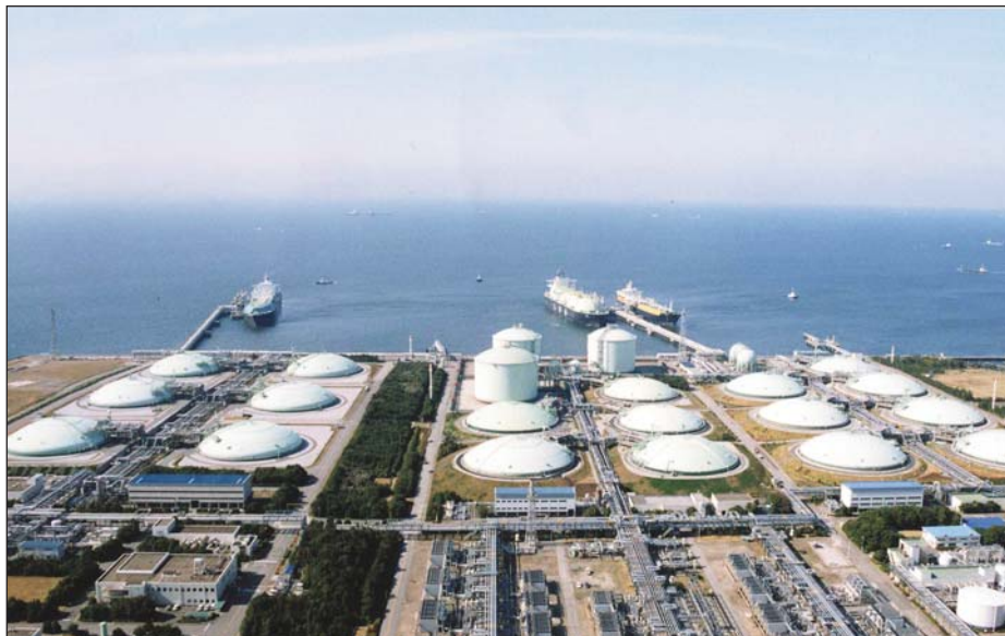
The Sodegaura LNG receiving terminal on Tokyo Bay opened in 1973 and is owned by Tokyo Gas and Tokyo Electric Power. It's among the largest LNG import terminals in the world, with an annual capacity of almost 30 million tons of LNG (1.5 trillion cubic feet of gas).
