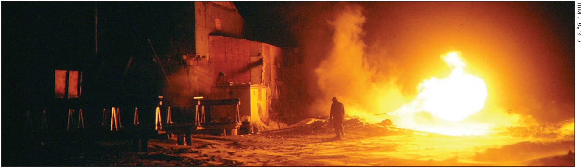
Workers flared the first gas flow from the Ivishak (Sadlerochit) Formation reservoir during Drill Stem Test No. 2 of the Prudhoe Bay State No. 1 well on Dec. 27, 1967. No oil flowed to the surface during the test, but natural gas flowed from the well with a rumble and roar that sounded like a jet plane overhead.
