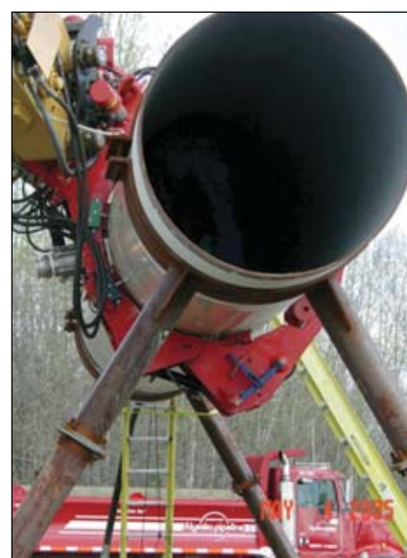
The clamp is the invention of Alyeska and Fairbanks engineering firms, which worked on the device after a man shot the pipeline with a high-powered rifle in 2001, causing a $20 million cleanup bill.
