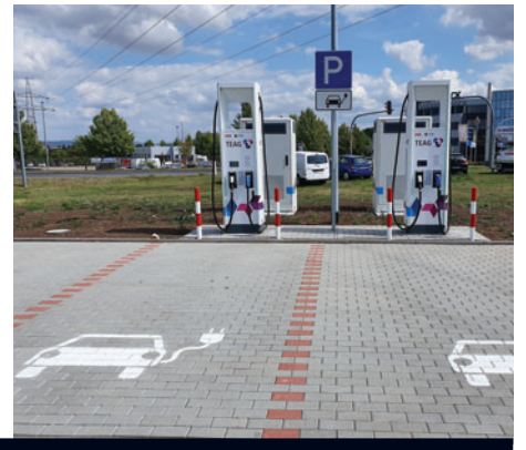
page 5 EV charging stations planned for AK road system; Cantwell online
