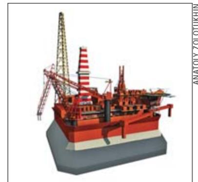
A gravity-based production and accommodation structure of the type to be installed in Russia's Prirazomlnoye field requires a large towing draft
