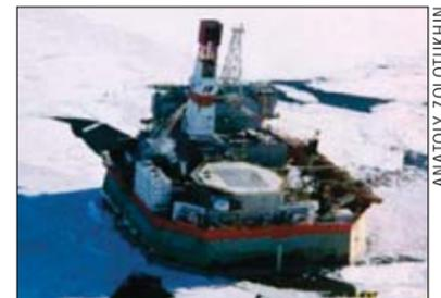
The massively strong Molikpak steel caisson structure that forms the producing Vityaz platform at Sakhalin
