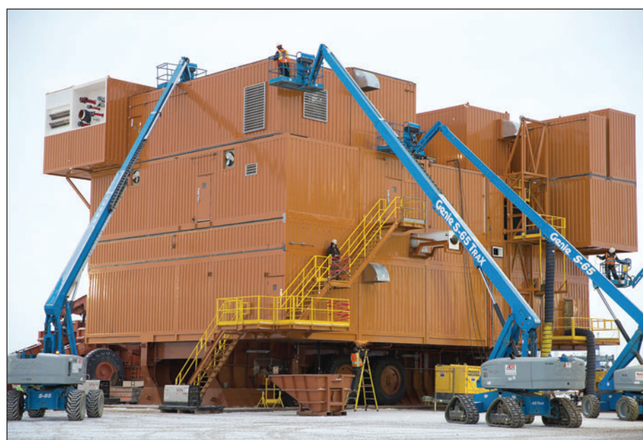
Four forklift man baskets supporting work on one ERD rig module in Deadhorse.
