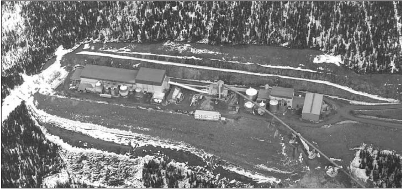
Ore from the high-grade Pogo gold mine is transported via a 2,500-foot long conveyor from the 1690 portal (where the photo was taken) to the surface mill (shown).
